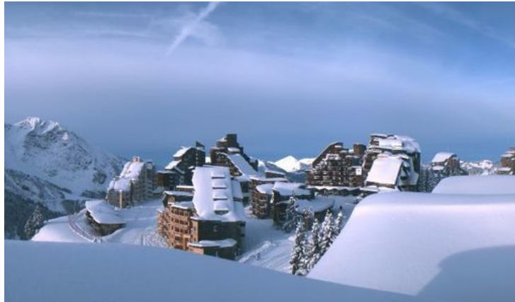
Excellent snow conditions in the Portes du Soleil. This is Avoriaz - Photo: avoriaz.com
